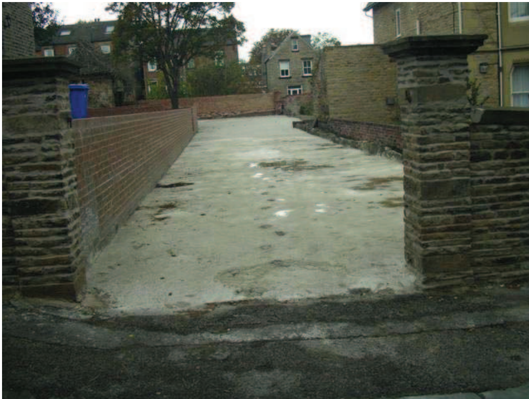
Photo of Concrete Hardsurfacing
